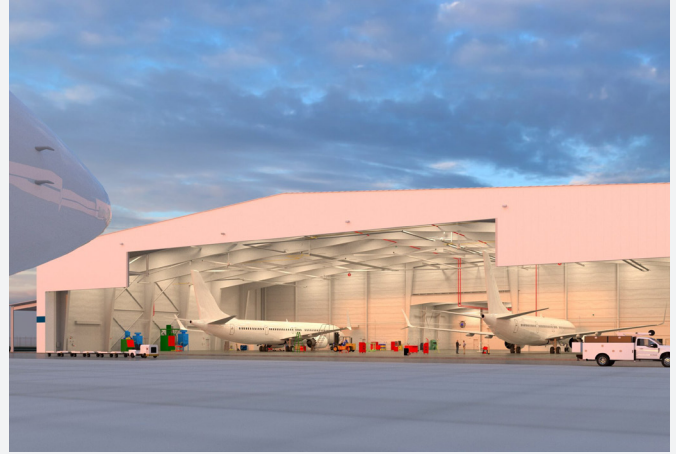
AMERICAN AIRLINES MAINTENANCE BASE Tulsa is home to the world's largest commercial aviation maintenance facility and was recently awarded $22 million from the State of Oklahoma.
