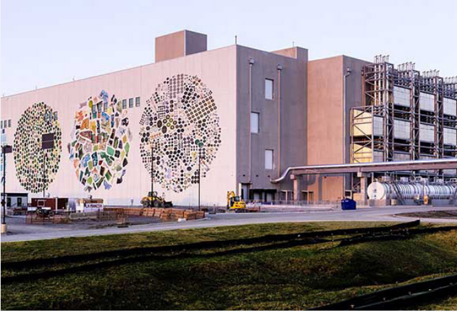
GOOGLE SERVER FARM Google's data center facility 45 minutes northeast of Warren Place citing the "right combination of energy infrastructure, developable land and available workforce."
