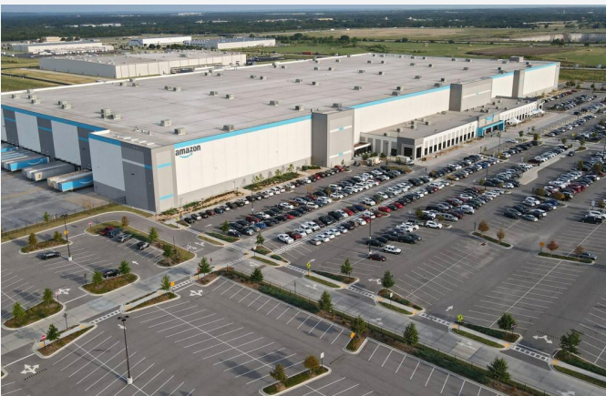
AMAZON FULFILLMENT CENTER Amazon opened a 2.6 million SF fulfillment center that employs 3,000 people.
